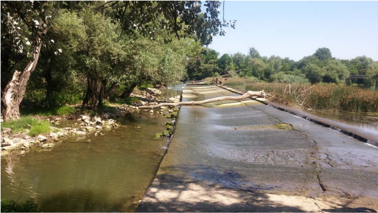
Figure 3. Drop structure (the picture is taken from the left bank, looking towards the right bank)
