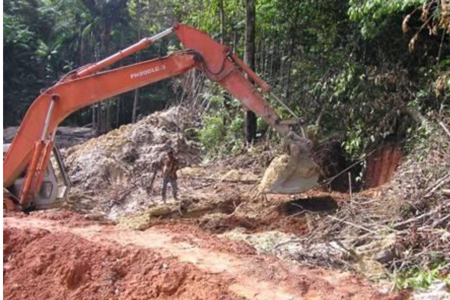
FRAME 3: STRIPPING OF TOPSOIL IN NIEUW KOFFIE KAMP
