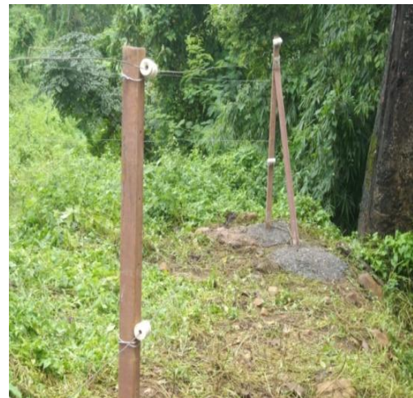
Solar electric fencing
