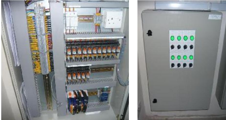
Figure 12: PLC on DX units
