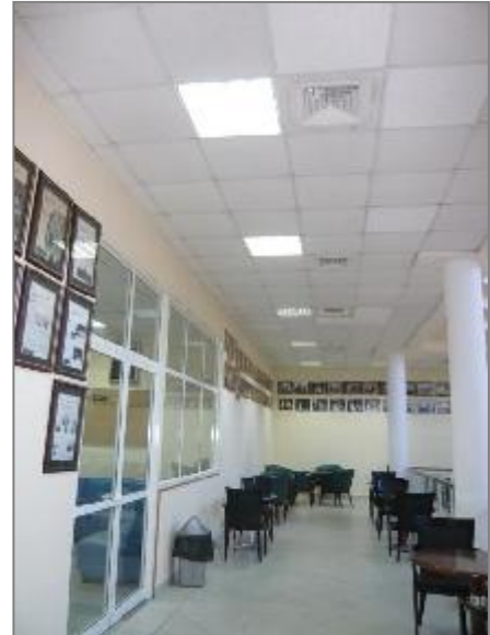
Figure 15: A corridor after the removal of extra light fixtures
