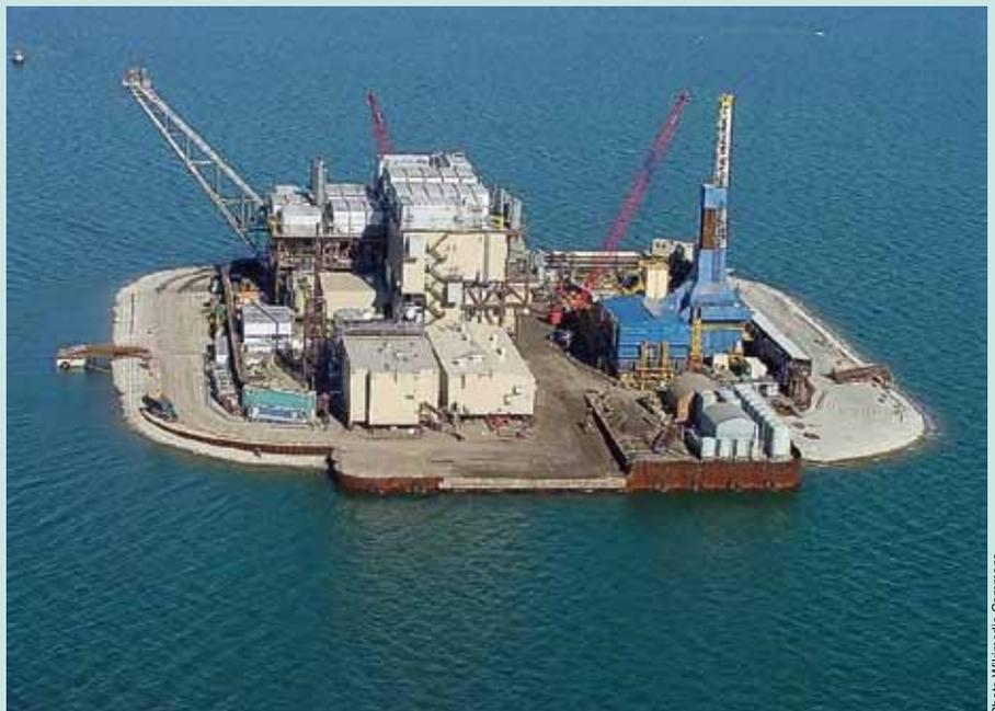
*Much of the Arctic is opening up to new human activity, including offshore oil and gas development. Here Northstar Island, an oil and gas drilling site built up as an artificial island in the Beaufort Sea north of Alaska.*
