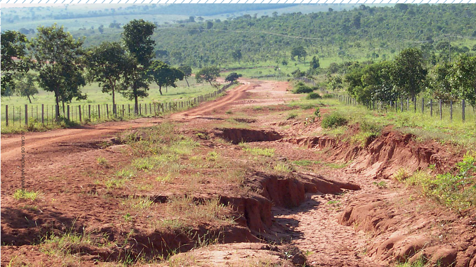
Soil erosion caused by road-building in the Paraguay river basin.
