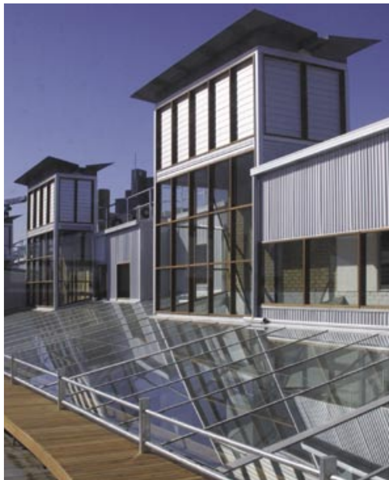
60L - Improved building design and solar chimney
