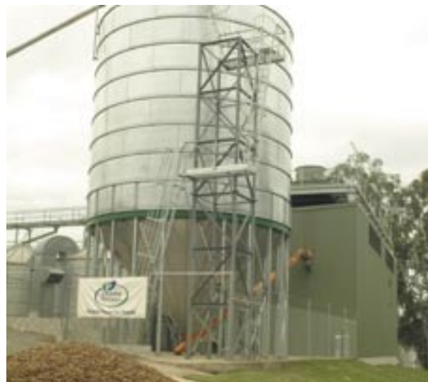
Use of waste macadamia nut shells as biomass fuel
