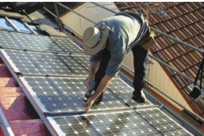
Installation of photovoltaic roof tiles
