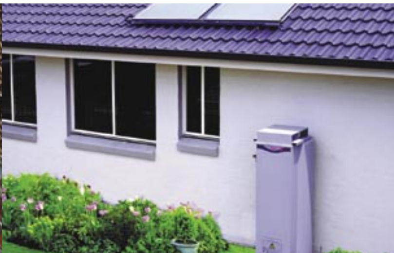
Solar and gas hot water heating
