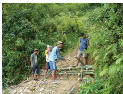
Live cuttings inserted between first and second layer stretchers
