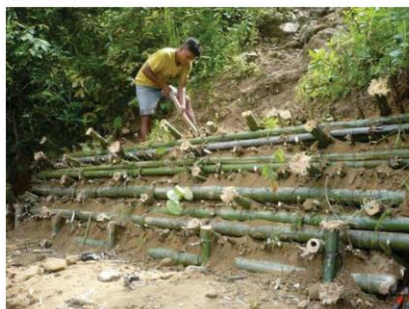
Five layers of crib wall construction completed to stabilize the base of the slope
