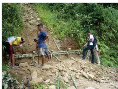
First layer of stretcher and header of the bamboo crib wall completed
