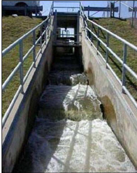
**Vertical-slot fish passage** is similar to a pool-and-weir system, except that each "dam" has a narrow slot in it near the channel wall. This allows fish to swim upstream without leaping over an obstacle. Vertical-slot fish passages also tend to handle reasonably well the seasonal fluctuation in water levels on each side of the barrier.
