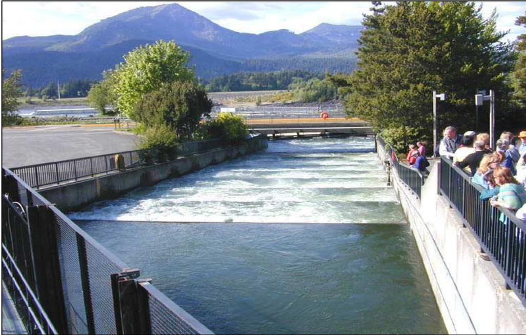
Fish ladders are very effective and relatively old device mentioned for first time in France during 17<sup>th</sup> century. One version of fish ladder was patented in 1837 by Richard McFarlan from Bathurst, New Brunswick who designed a fishway to bypass dam at his water-powered lumber mill. There are five main types of fishways: Rock-ramp fishway, Pool and weir, Vertical-slot fish passage, Baffle fishway and Fish elevator.
