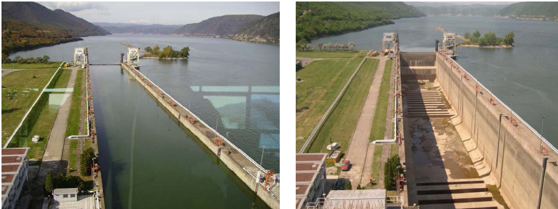
Figure 2.5 Djerdap 1 lock (Serbian side) full and empty (Source: Witteveen – Bos)
