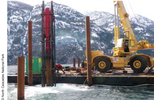
A bubble curtain being installed.
