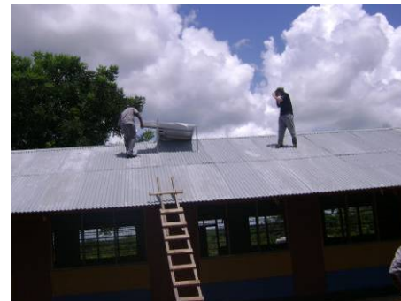
Installation of solar panels at secondary school © WWF - Cyprien
