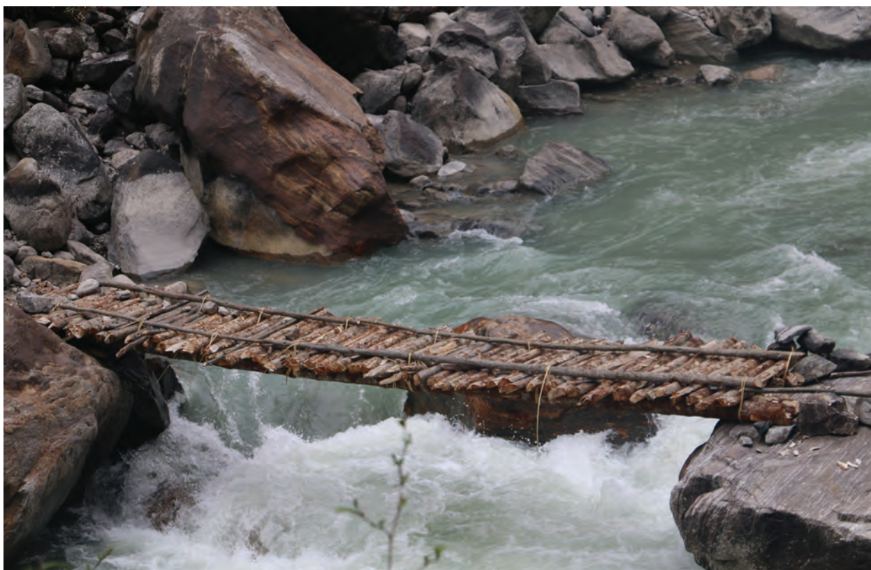
Wooden bridge installation to facilitate access as part of pasture land management interventions. © Deepak Upadhyaya / WWF Nepal
