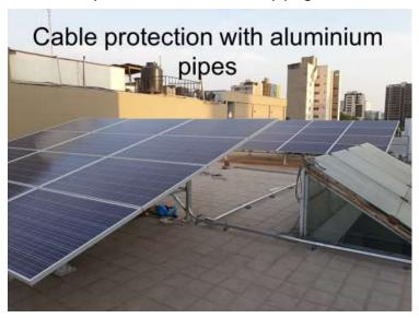
4) The solar cabling should be arrange so as to avoid electro-magnetic interference and induced overvoltage from nearby lightning strikes
