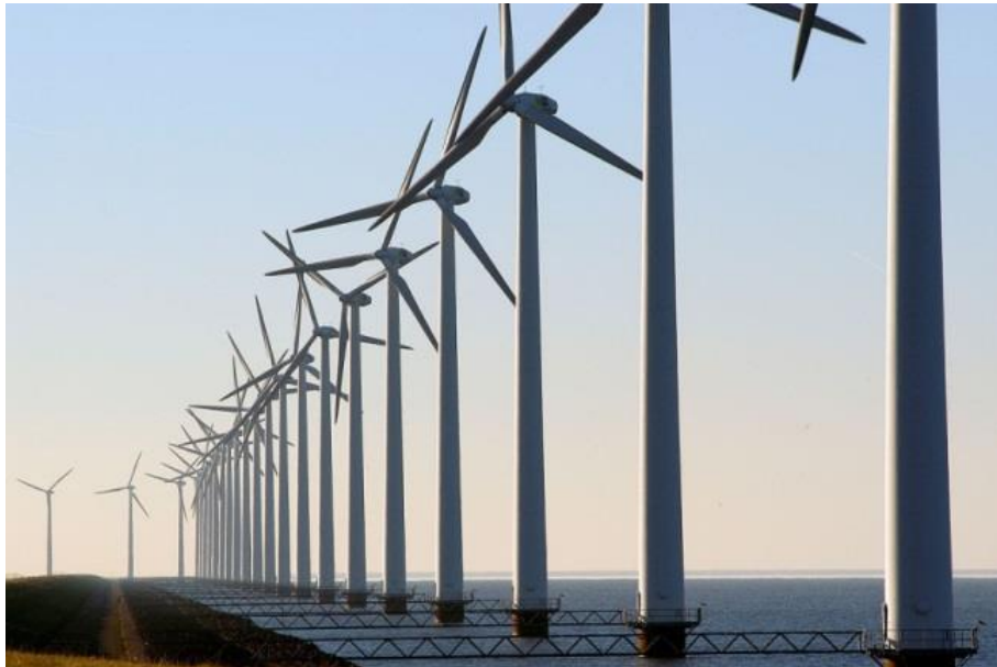
North Sea wind turbines, off the Netherlands. © Gunther / WWF
