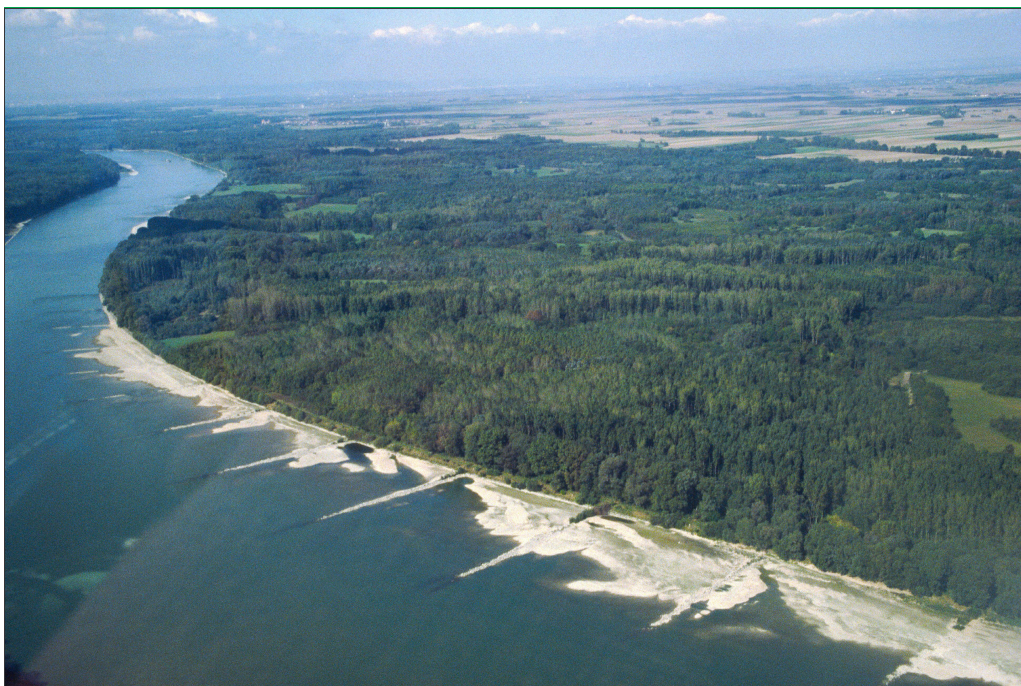
Fig. 4.2 Groynes along the Danube stretch in Austria. ( Photo credit: B. Lötsch )
