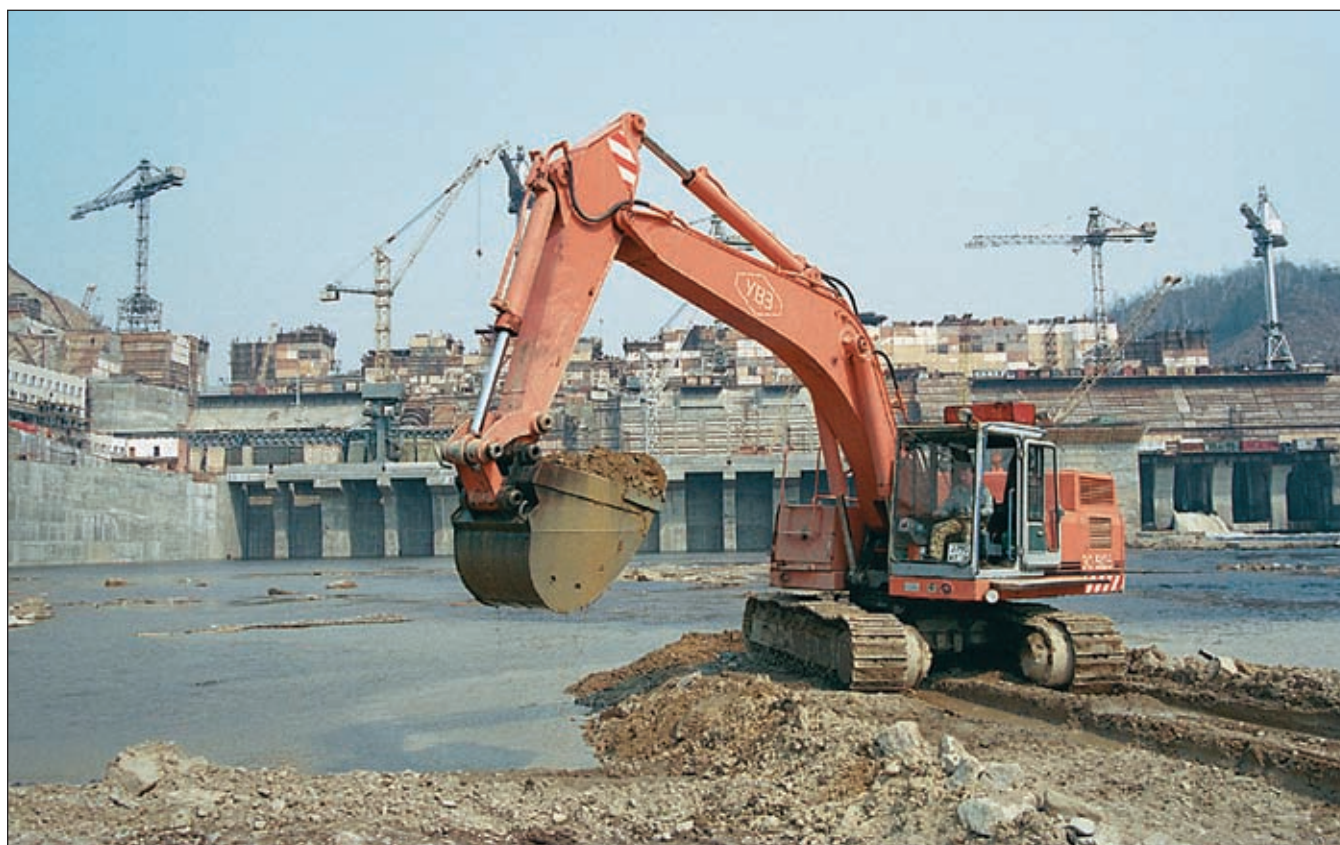
Construction of Bureya Hydropower Plant © WWF-Russia / Z. Taigi
