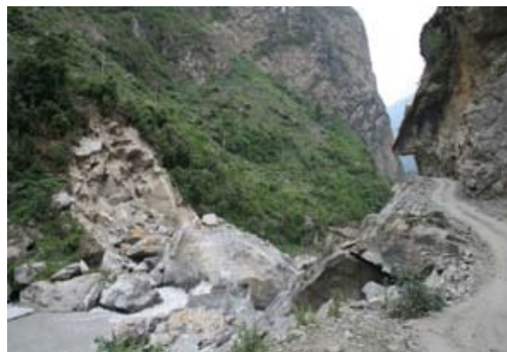
Figure 10: Massive pieces of rock deposited in the river channel along the Besishahar-Chame Road. Similar deposits consisting of large stones and/or smaller pebbles and rock fractions were observed at multiple points along the road
