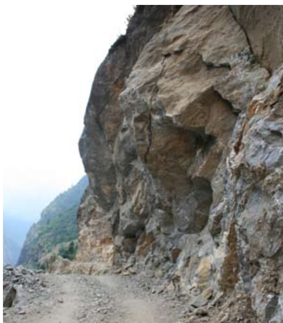
Figure 9: Unstable slopes and fissured landscape along Besishahar-Chame Road
