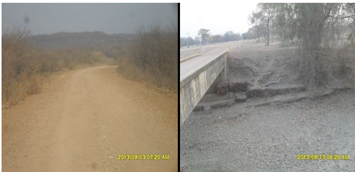
Fig 4.24 Typical gravel roads in Gokwe North (Threatened by gullies)
