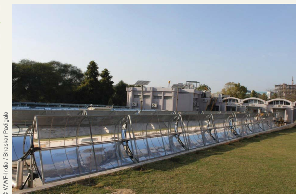
FIGURE 2.19 PTC-Based Solar Air-Conditioning System at SEC, Gurgaon
