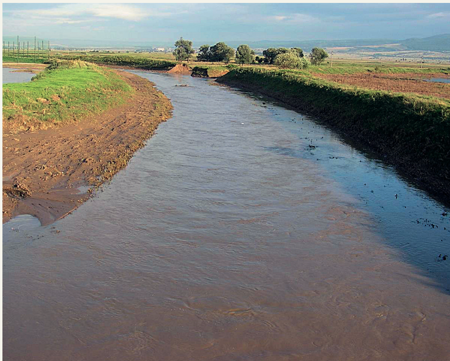
Fig. 15. Straightening of the Lesnovksa River in Ravno Pole
